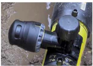
The PlassGas reuseable solution is specifically designed for purge points and temporary bypass applications.
